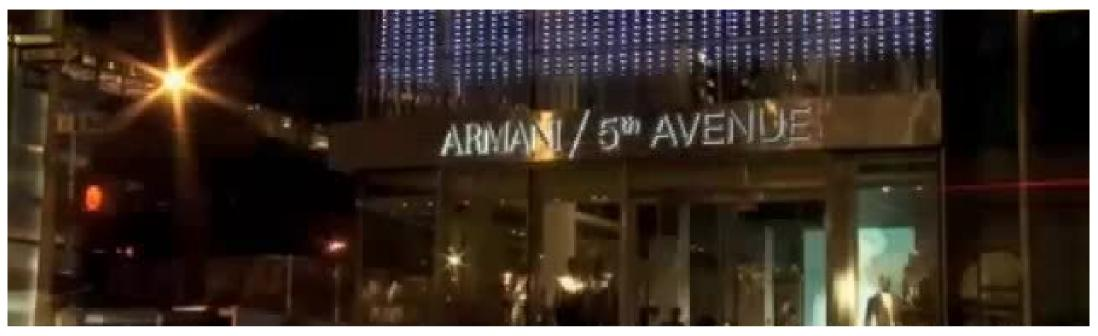
To preserve the transparency and the artistic intention in respect of planning conditions for 5th Avenue, we developed a unique light façade from a series of vertical, mirror-polished bars that 'dissolve' into the architecture of the building and become increasingly sparse along the building's W56th Street Elevation.
